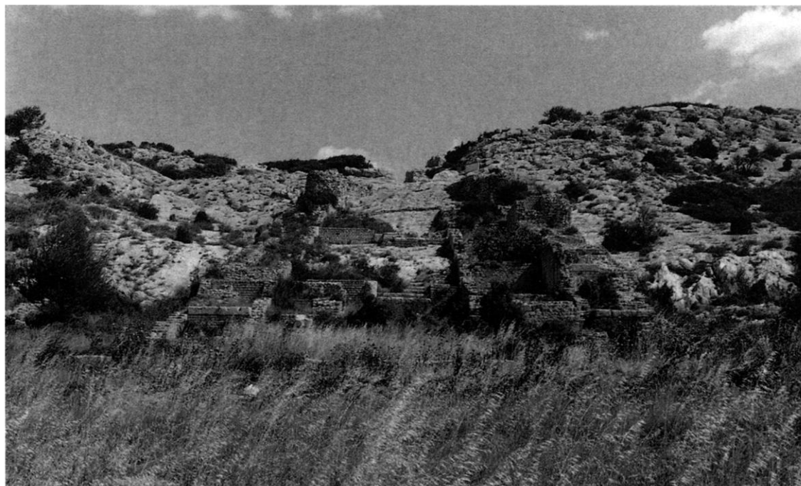
2. THE SECOND-CENTURY A.D. LARGE WATER-MILL COMPLEX AT BARBEGAL NEAR ARLES. THE AQUEDUCT ENTERING THROUGH THE ROCK-CUT GAP AT THE TOP OF THE RIDGE DIVIDES INTO TWO MILL-RACES, EACH OF WHICH DROVE EIGHT OVERSHOT WHEELS. Photo: A. Wilson
